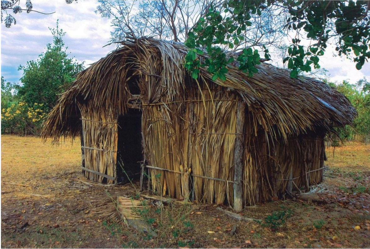
Figure5–Hut made from palm straw and earth, at the edge of a vereda. Municipality of Bonito de Minas in Minas Gerais.Source: Boaventura (2007, page 153)
